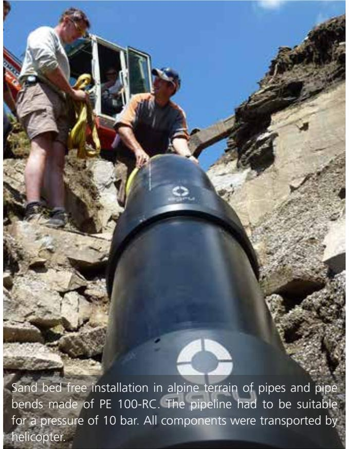
Sand bed free installation in alpine terrain of pipes and pipe bends made of PE 100-RC. The pipeline had to be suitable for a pressure of 10 bar. All components were transported by helicopter.
