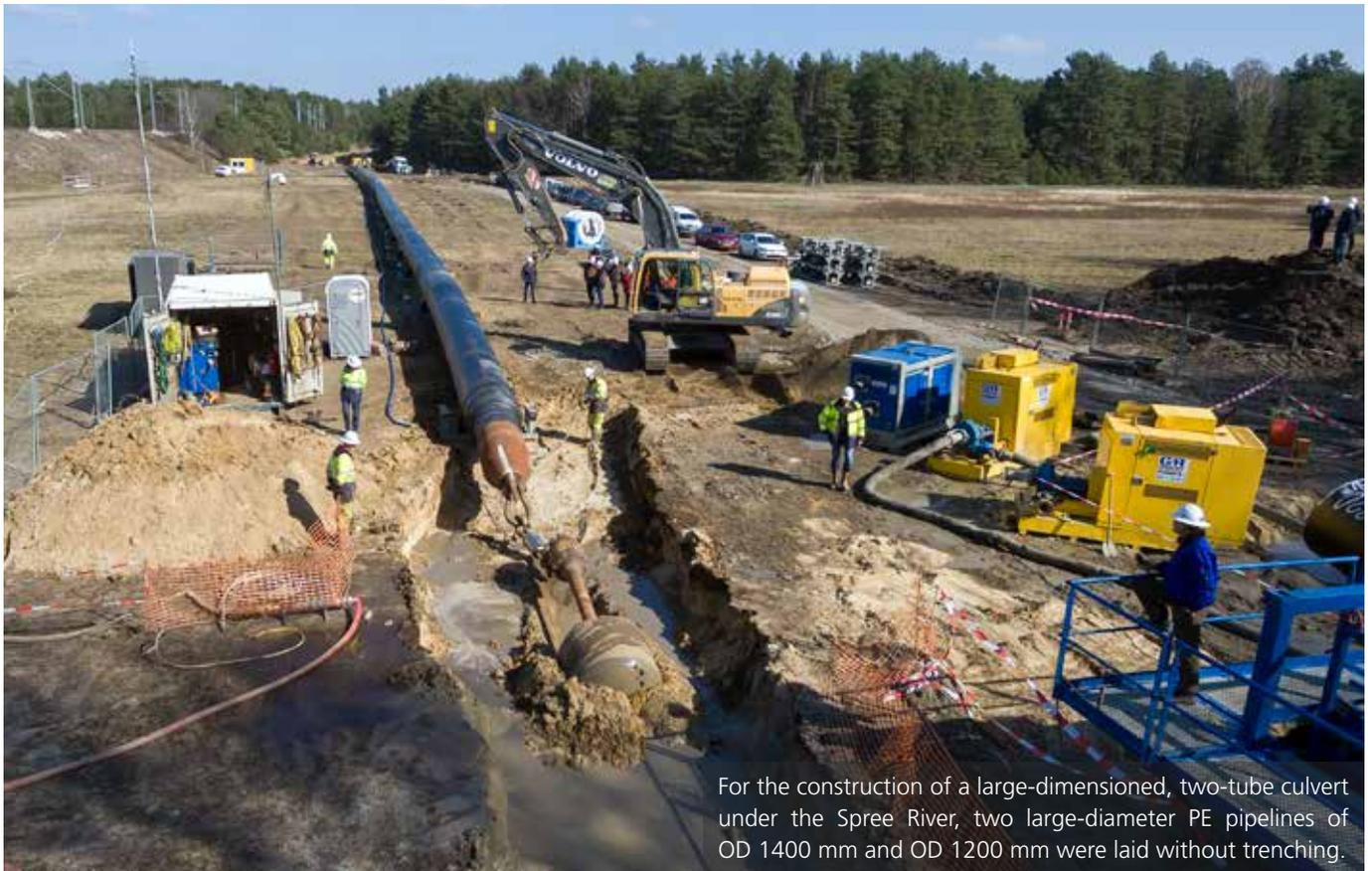
For the construction of a large-dimensioned, two-tube culvert under the Spree River, two large-diameter PE pipelines of OD 1400 mm and OD 1200 mm were laid without trenching.
