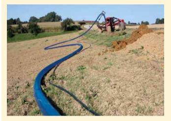
The coloured signal layer denotes the application - here a potable water line.
