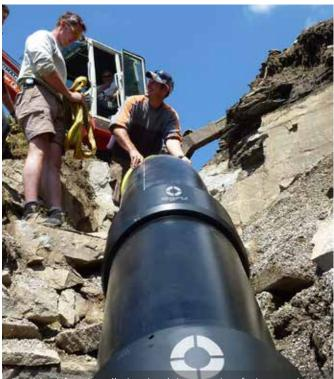
Sand bed free installation in alpine terrain of pipes and pipe bends made of PE 100-RC. The pipeline had to be suitable for a pressure of 10 bar. All components were transported by helicopter.
